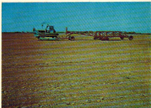
Soil levelling by П-4 leveller
