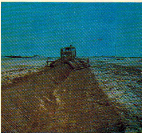
Making protective mounds by BY-0,7 mound-making machine
