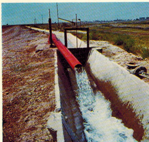
Vertical drainage providing pumped water for irrigation
