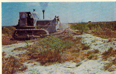
Cutting knolls and shrubs by C-100 bulldozer
