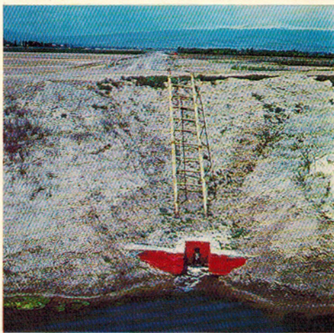
Closed horizontal drainage
