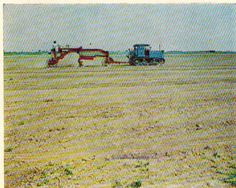
Primary soil levelling by Д-20Б grader
